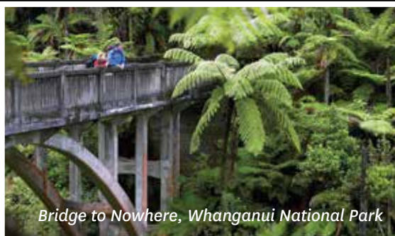
Bridge to Nowhere, Whanganui National Park
